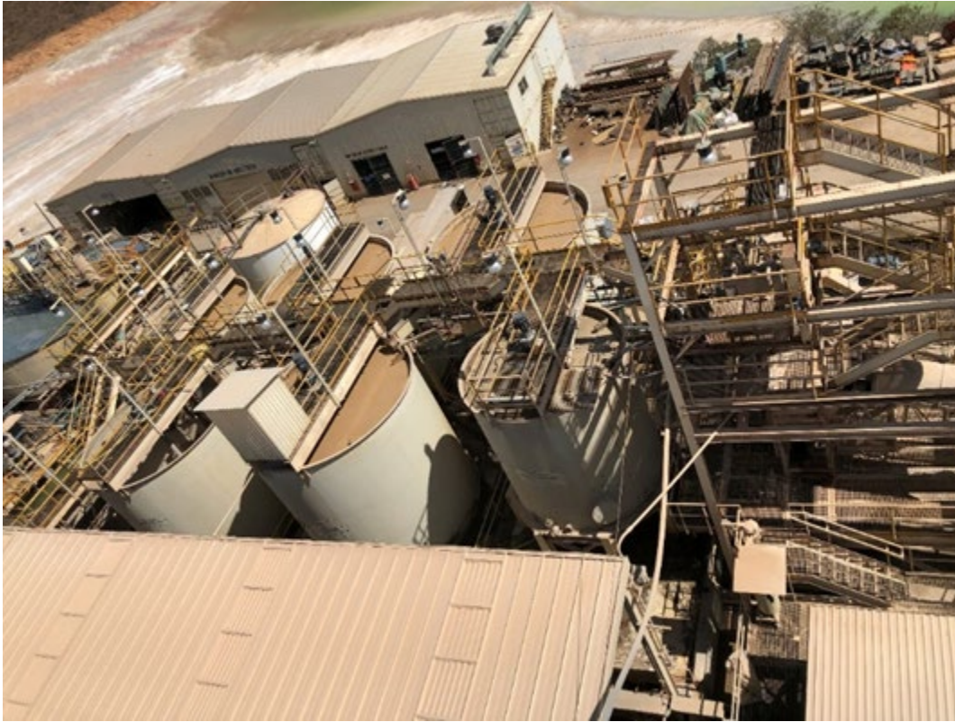
Figure 17-5: Agitated Leach Circuit of the DDGM Processing Facility
